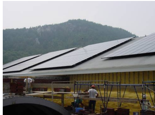
A 56 kW solar photovoltaic array was installed on this middle school's south-facing roof. The array will supply 9.9% of the school's as-designed energy needs.
