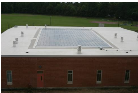
A 34 kW solar photovoltaic array was installed on the roof of this school's swimming pool building. The array supplies 2.3% of the school's as-designed energy needs.
