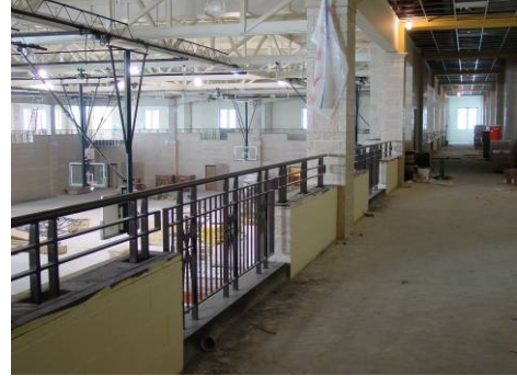
An elevated walking track surrounds this gymnasium. Citizens may be able to use it at times throughout the day as allowed by the school district.
